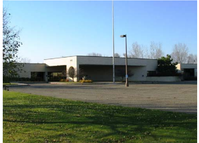
Future home of the District and Community Services Center, 1415 81st Street, Spring Lake Park
